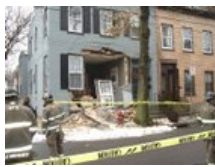
Front wall of Stockade home collapses
